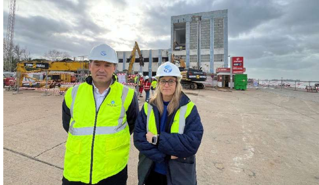
The President of the Port of Huelva, Alberto Santana, and the Head of the Infrastructure Department, Guadalupe Díaz, during the start of the demolition of the Expofrisa warehouses.
