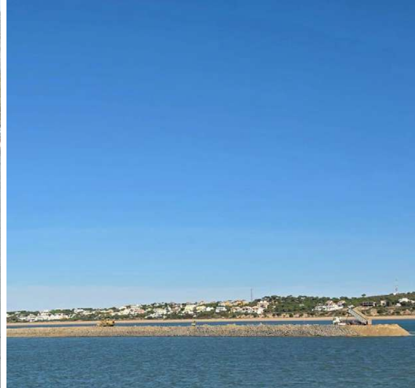
Site No. 4 Phase 2 (during construction).
