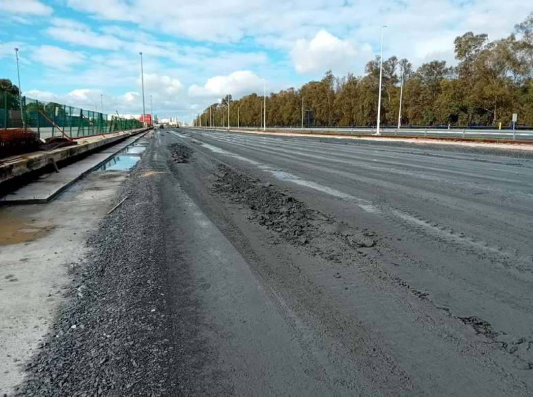
Railway terminal expansion (during construction).
