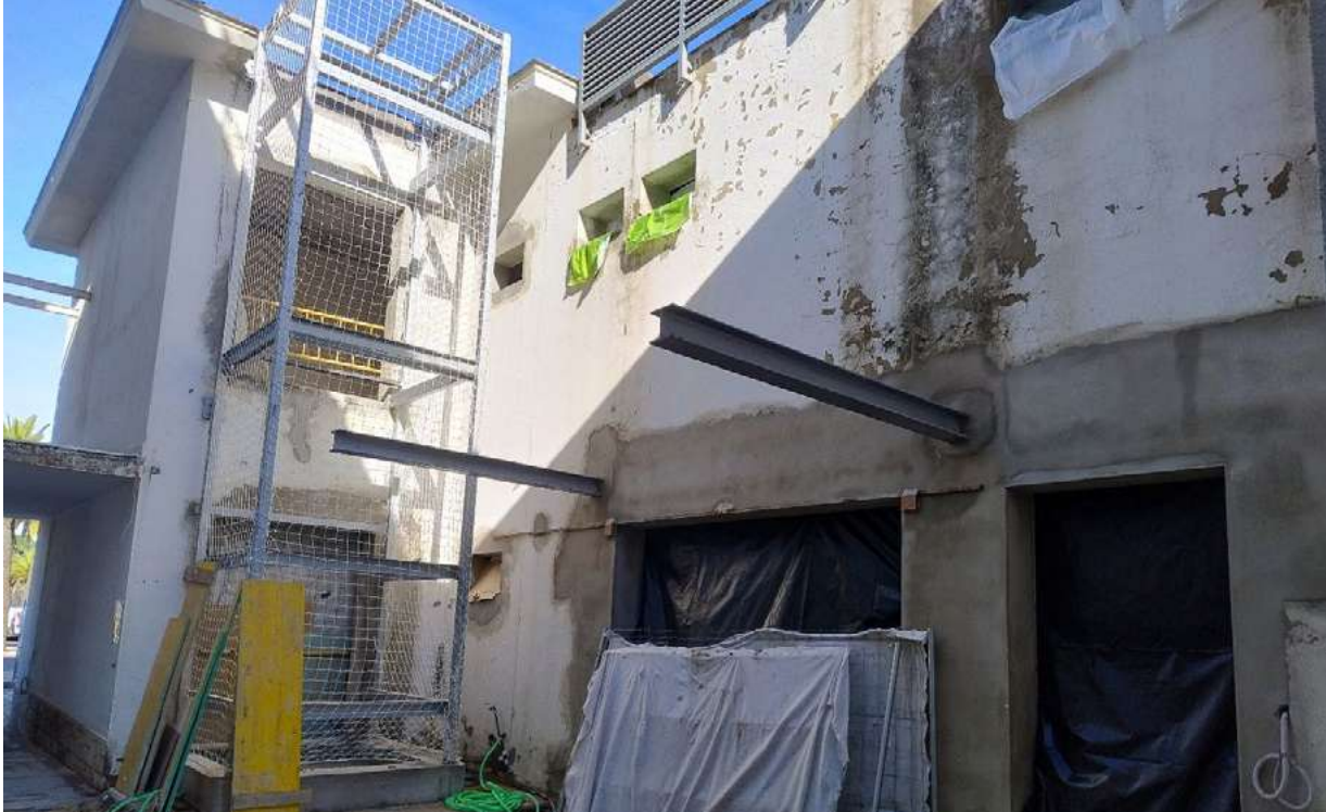
Refurbishment of the Estihuelva building (during works).
