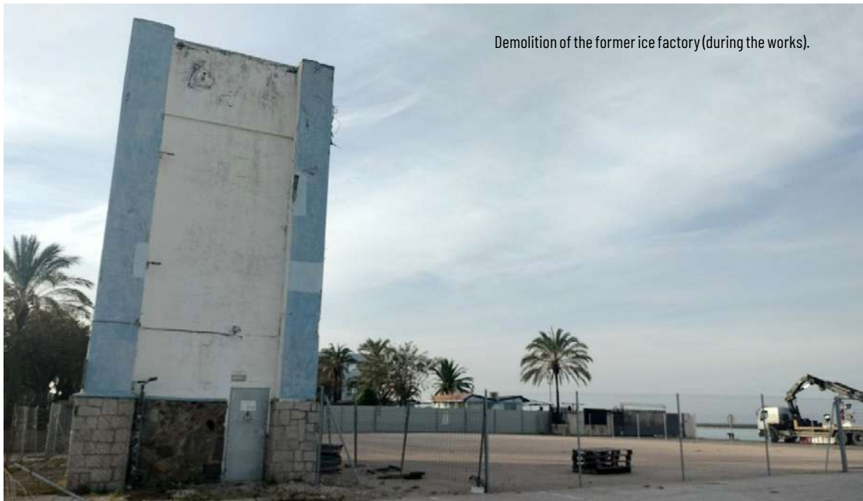
Cold pipeline rack (during construction),
