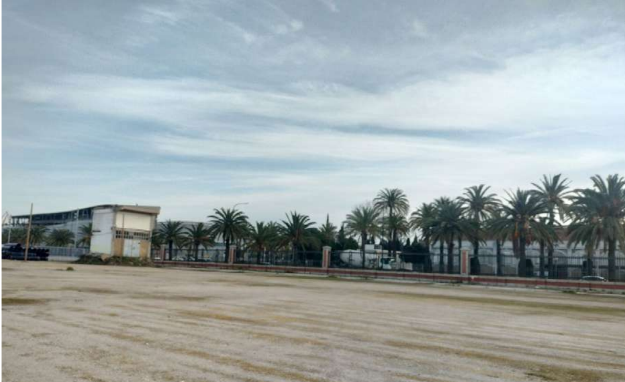
Demolition of the final section (during the works).
